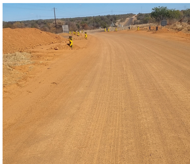
Photo: Road work
